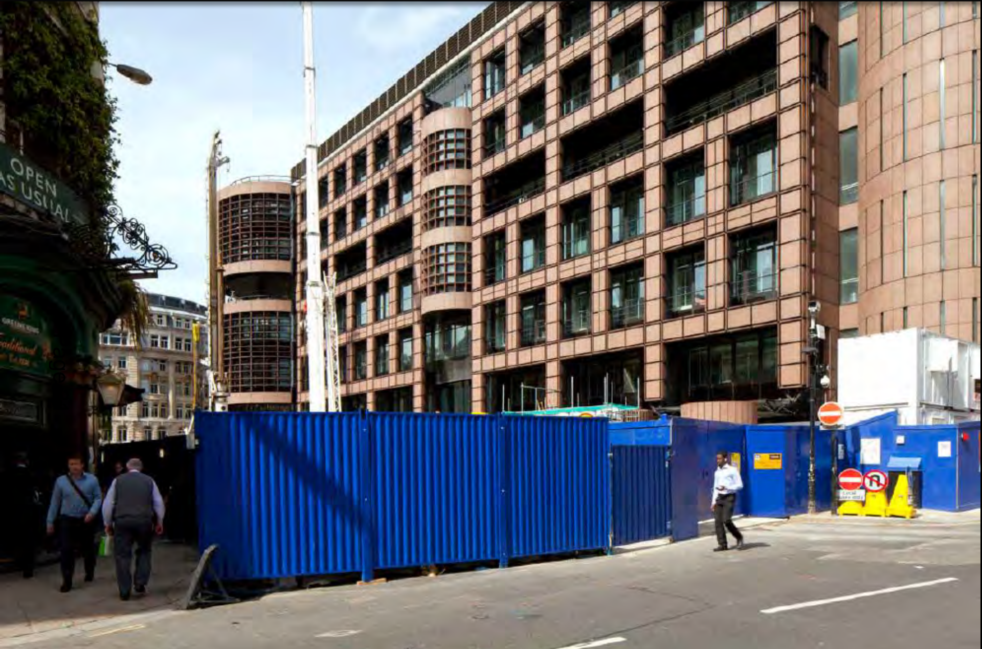
Existing view from Liverpool Street looking north-west
