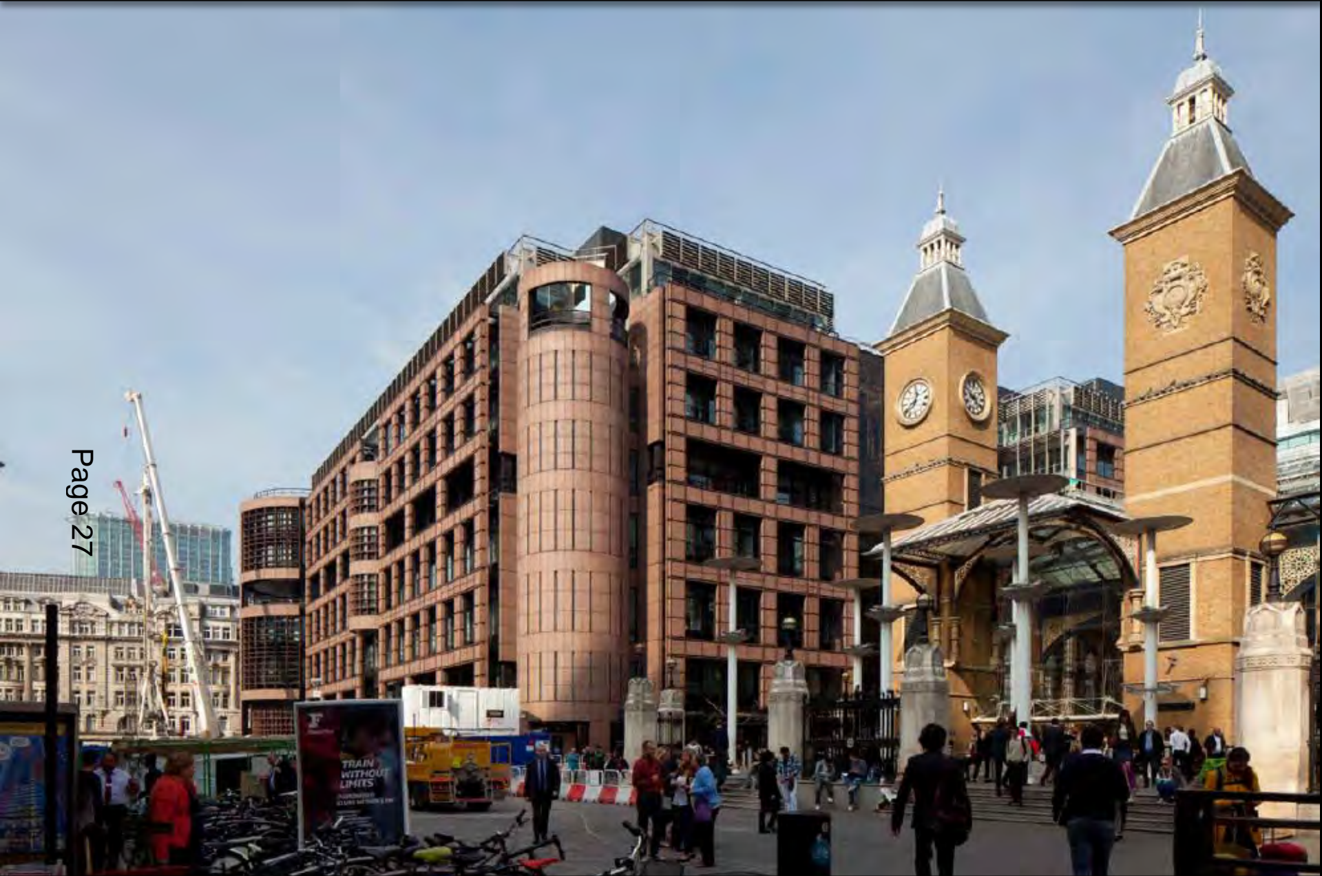
Existing view from Liverpool Street looking north-west
