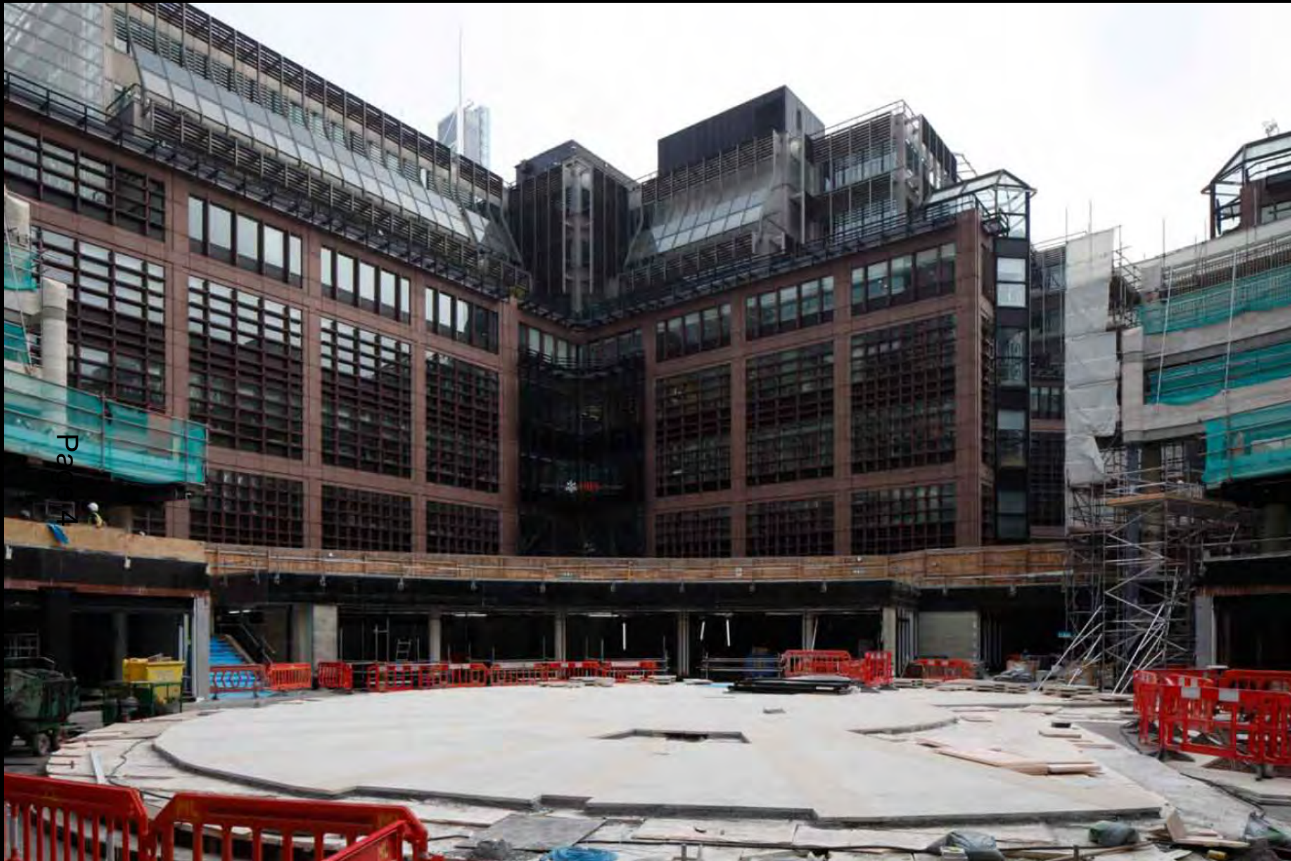
View south-east from Broadgate Circle
